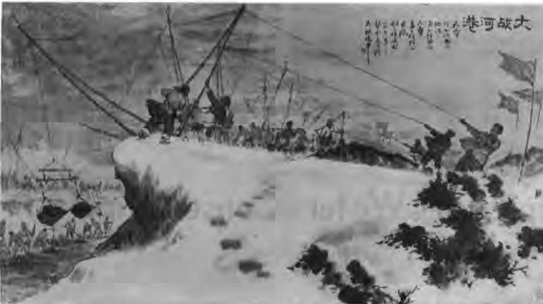
Dredging the canal
